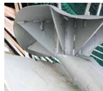
Figure 9: Mushroom head of the stainless steel structure. Bent over the centre column and deformed. On top of the steel structure are visible the sticks that have been used as guidance for the 52 belts laid over the mushroom head
