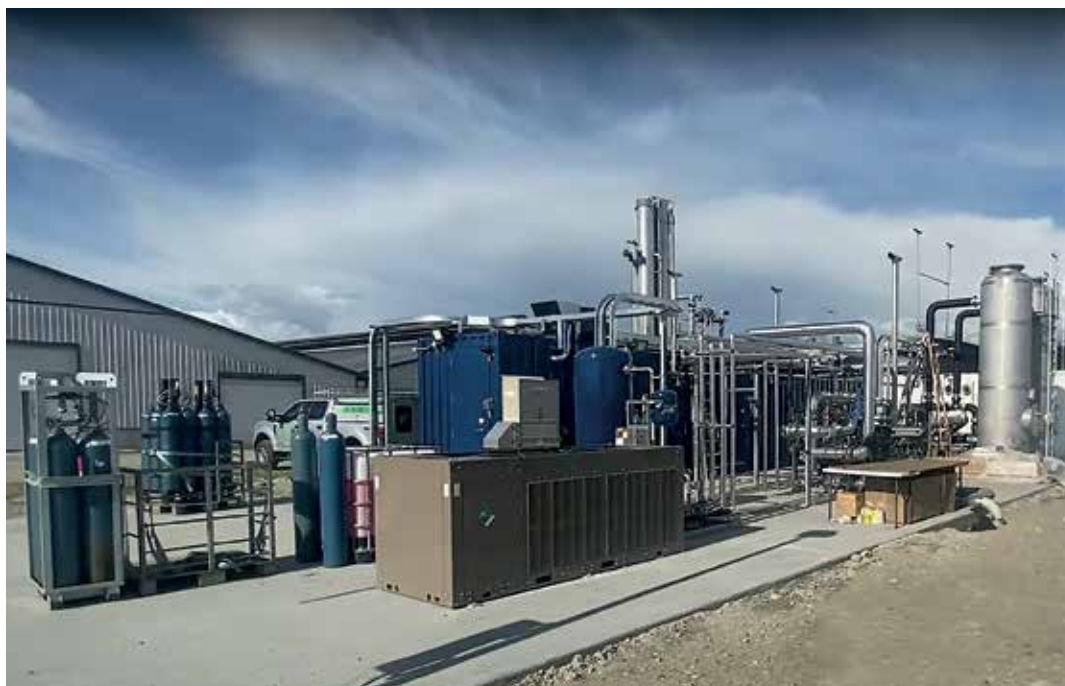
A mid-size dairy farm in British Columbia replaces a water wash system with DMT's Carborex® MS, a membrane separation system, to extract CO 2 from the methane (CH 4 ) stream
