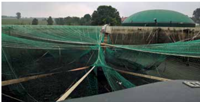
Figure 1: Looking into the digestate storage tank. The gas holder roof membranes already removed. Belts, net, crooked centre column. Background right hand side: secondary digester tank with double membrane gas holder roof
