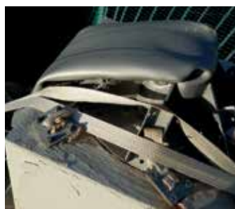
Figure 7: View on the top of the centre column. Massively deformed stainless steel construction. 'Mushroom' bent over to the left. Cracked belt visible on top left of the concrete head of the column
