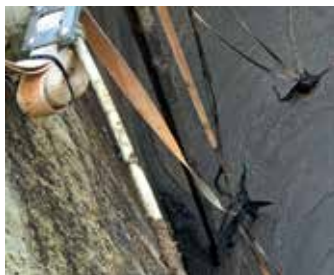
Figure 4: Belts wound around submerged mixer. Top left hand side: belt package with cable tie. For more details details, see Figure 5
