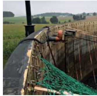
Figure 3: Tank wall with belts still fixed at the wall. Most belts in this area cracked and hanging into the digestate. Left hand side: overpressure/vacuum valve with related outflow pipe (in orange) and mast for submerged mixer next to it
