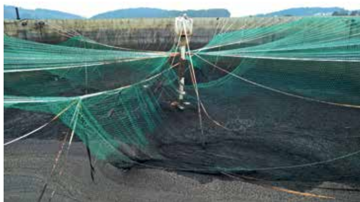
Figure 2: Fully visible centre column, crooked, with massively deformed stainless steel construction on top. Tank still filled with about 1 m of digestate. Net and some belts lying in the digestate
