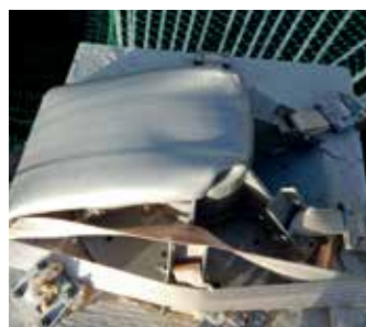
Figure 8: Fixing of the 'additional belts' that have been used for mounting the belt and membranes of the roof structure. Visible are five such belt connections to the stainless steel construction with the sixth one being buried underneath the bent steel structure
